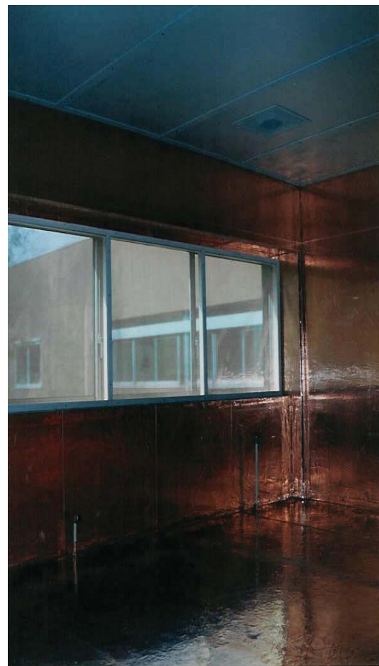
Screened windows for daylight accession
